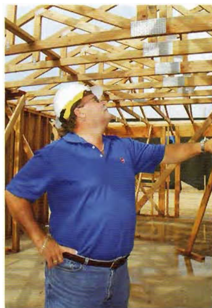
Gentry's Bob Kayser conducts inspections at the Kanehili neighborhood in West Oahu.
